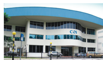
CEI Contract Manufacturing Limited 2, Ang Mo Kio Avenue 12 Singapore 569707
